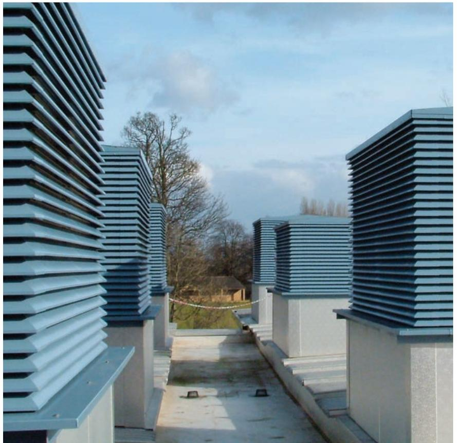
*Pre-assembled 3UL louvre turrets on top of natural vent shafts.*
