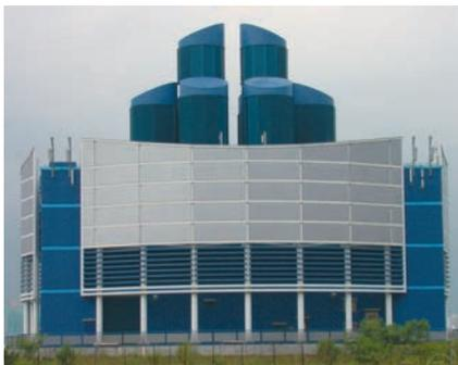
*Triple bank faceted circular louvre installed to handle the high air volumes required and to provide maximum rain protection even in typhoon conditions.*
