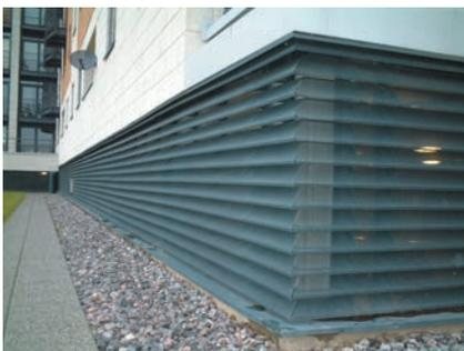
Perforated louvre allows additional daylight into this partially underground car park.
