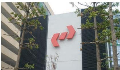
Colt inverted Universal Louvre is used extensively for this new underground station to provide high volume airflow with rain defence for plant rooms, entrances, vent shafts and external decoration.
