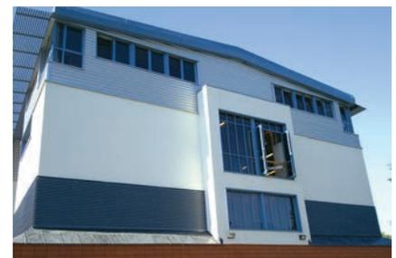
ERD louvre panels on the plant room, and Solarfin solar shading panels.
