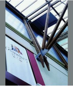
Gunwharf Quays, Portsmouth. Colt OPV controlled Seefires installed into a Colt roof glazing system. Fixed glass smoke curtains are also installed at high level.
